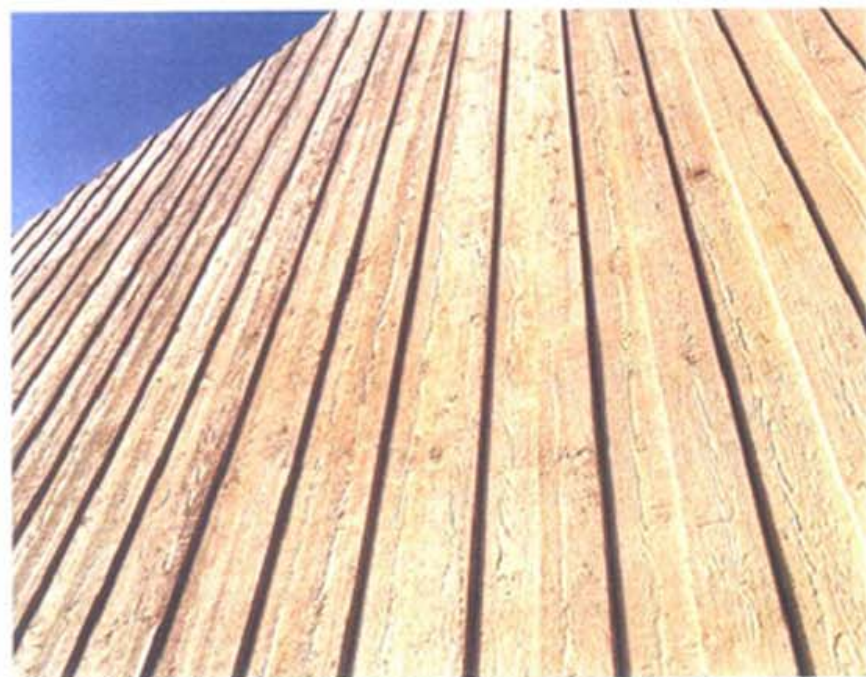
Sawn-board finish using rubberised form liner
