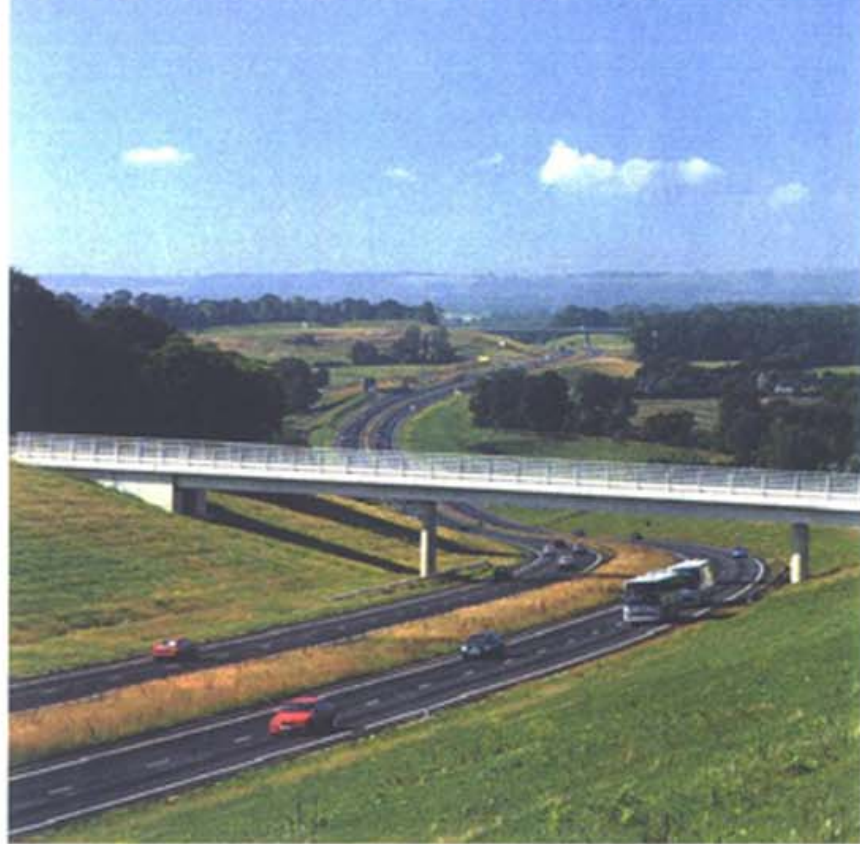
General view of the completed scheme meandering through the Berkshire countryside.
